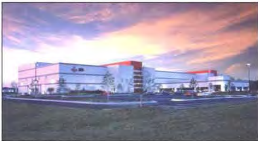
The AIDA plant in Dayton, Ohio— one of the world's most advanced press manufacturing facilities.
