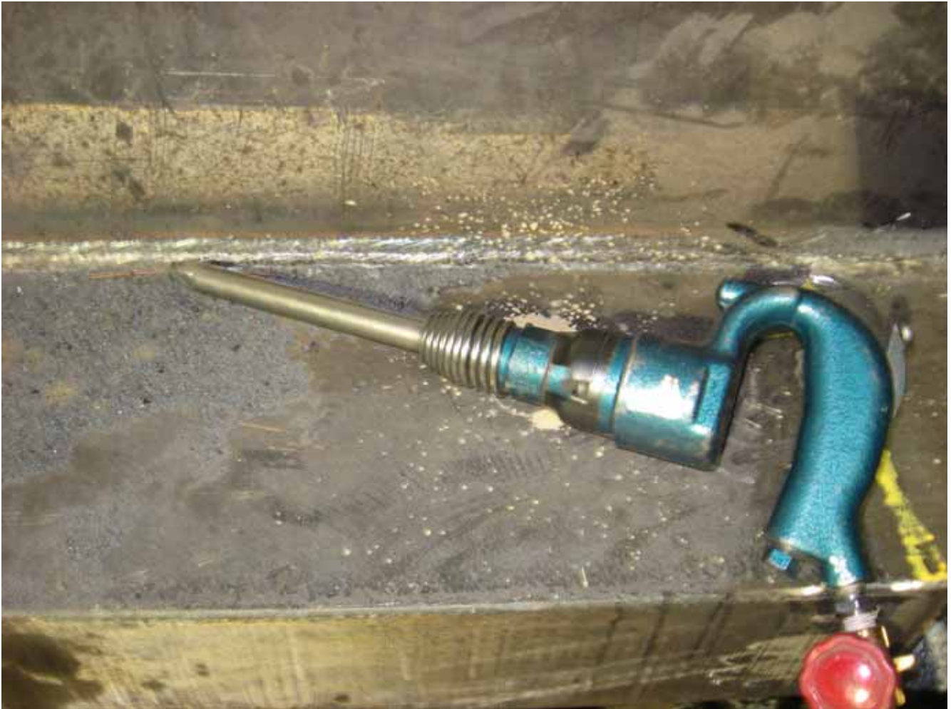
Air hammer for penning the weld
