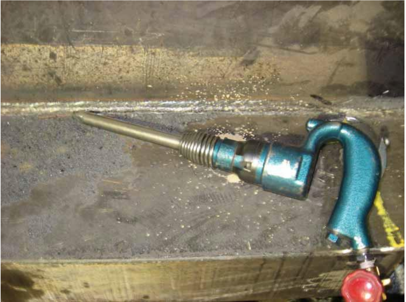
Air hammer for penning the weld
