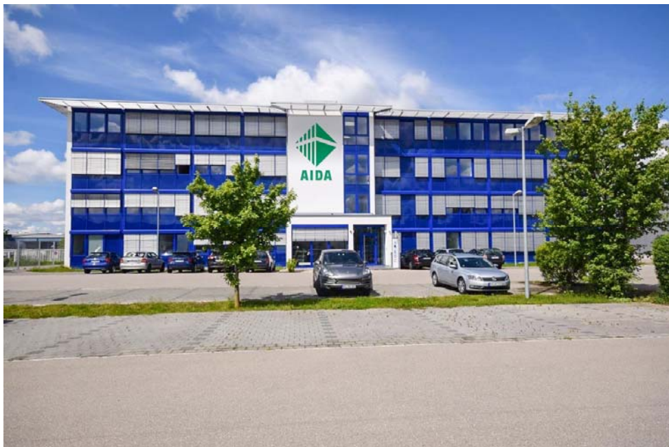
Photo#2: AIDA EUROPE GmbH new office building in Weingarten, Germany
